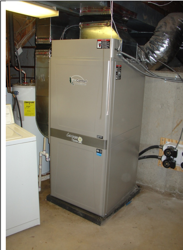
The new Heat Pump Furnace replaces the original natural gas burning furnace. Because the GeoExchange technology does not burn any fuel (fossil or bio), there is no need for an exhaust flue / chimney. So much for Santa Claus, sorry kids.
