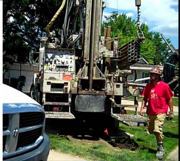
With the rig in place and erected, checkout proceeds
