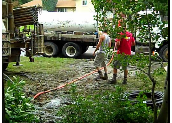
The last step for the drilling crew is to "grout" the tubing. A bentonite clay / sand mixture is used as the grout to fill in the space around the tubing and provide a heat transfer path between the tubing and the ground. The orange pipe is inserted down the well to the bottom and the grout is injected – the orange hose is then slowly pulled upward as the hole fills with the grout – eventually the grout starts oozing out the top of the hole.
