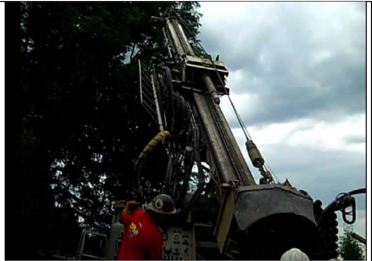
After the hole has been drilled, the boom is lowered - notice we provided some trees to make this a bit more challenging.
