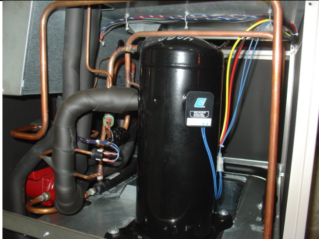
The compressor for the heat pump is directly below the blower assembly.
