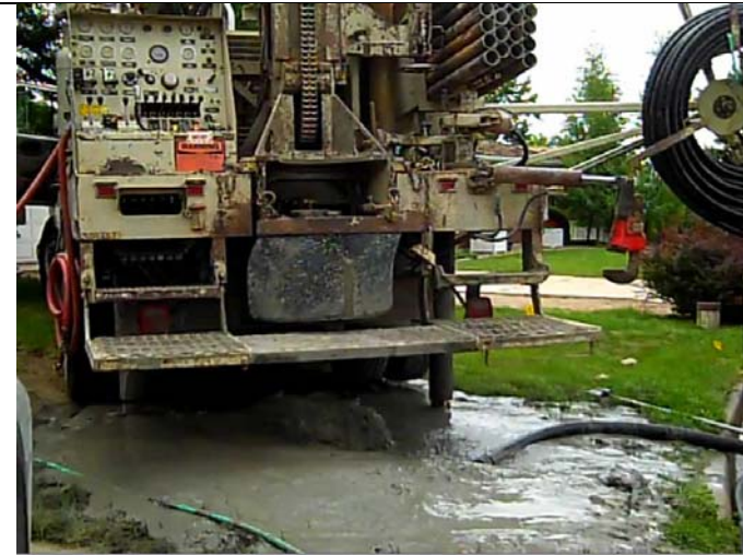
After about an hour and half, the drill bit had penetrated to about 300 feet (using 15 of the 20 foot sections of drill pipe). The drill pipe/bit has been raised back out of the hole. Now it's just a matter of dealing with the drilling mud.
