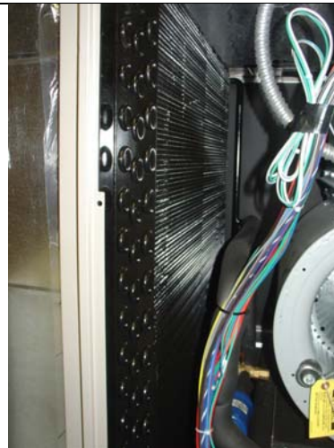
A closer look shows that the "cold air" is pulled through a heat exchange radiator by the blower assembly. The radiator temperature is controlled by the heat pump compressor – notice there are three layers of small black coils looping around the radiator. The fluid circulating in these small tubes is either hot or cold depending on how the heat pump is being driven – i.e. whether the house is being heated or cooled.
