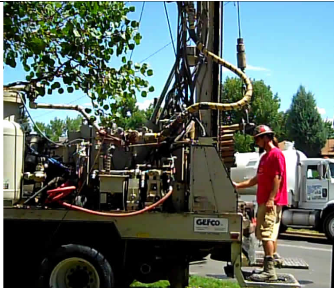
Last minute checks as drilling is about to begin
