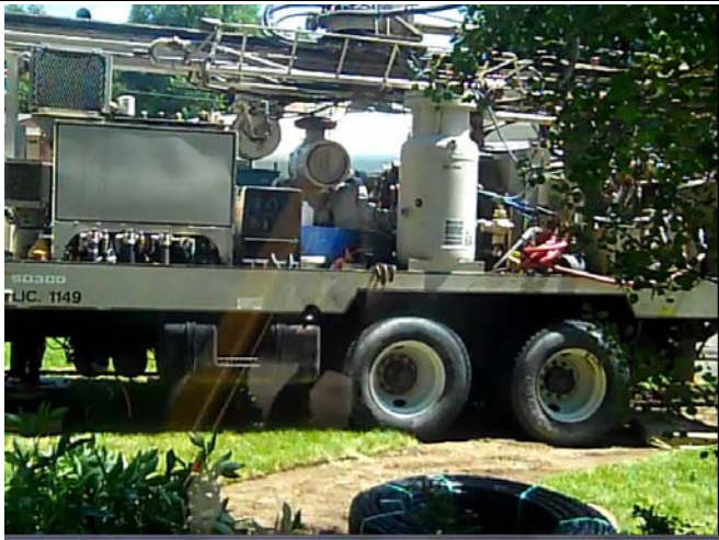
If you decide to install a vertical geothermal ground loop on your property, get mentally prepared for a drilling rig to show up in your yard. The strip of bare ground shows where we had stripped the sod between the locations of the two proposed "wells."
