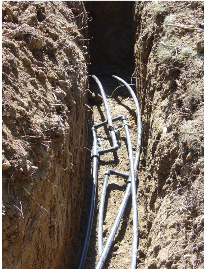
Manifold in place, soon to be tested for leaks and then the trench will be backfilled.
