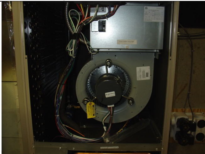
The Heat Pump Furnace assembly is much like a gas-fired furnace in that it uses the same cold and hot air ductwork, and a fan/blower to circulate cold and hot throughout the house. This photo with the furnace cover removed, shows the blower assembly where air from the "cold air" register enters on the left side and exits through the "hot air" plenum at the top of the photo.
