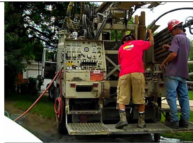
Before moving the drill rig, the 300 feet of double black plastic tubing is inserted down into the borehole from the spool to the right
