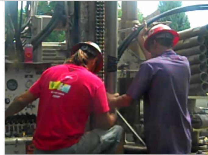
The black plastic is being inserted. On this hole, apparently material fell back into the bottom of the hole making it difficult to insert the last 25 feet of tubing. The tubing was taped to a section of drill pipe in an unsuccessful effort to drive it further down
