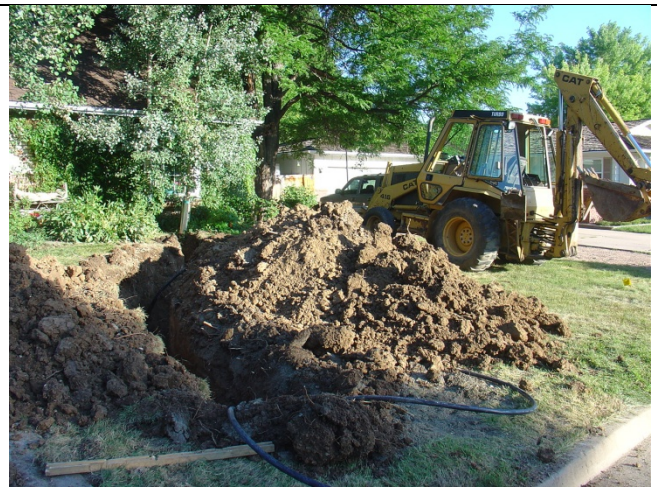
The scene after a few hours of work with the backhoe
