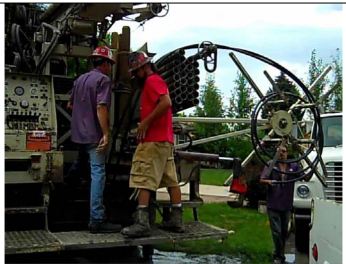
The black plastic 1" tubing is now in place. About 20 feet of excess tubing remains on the spool.
