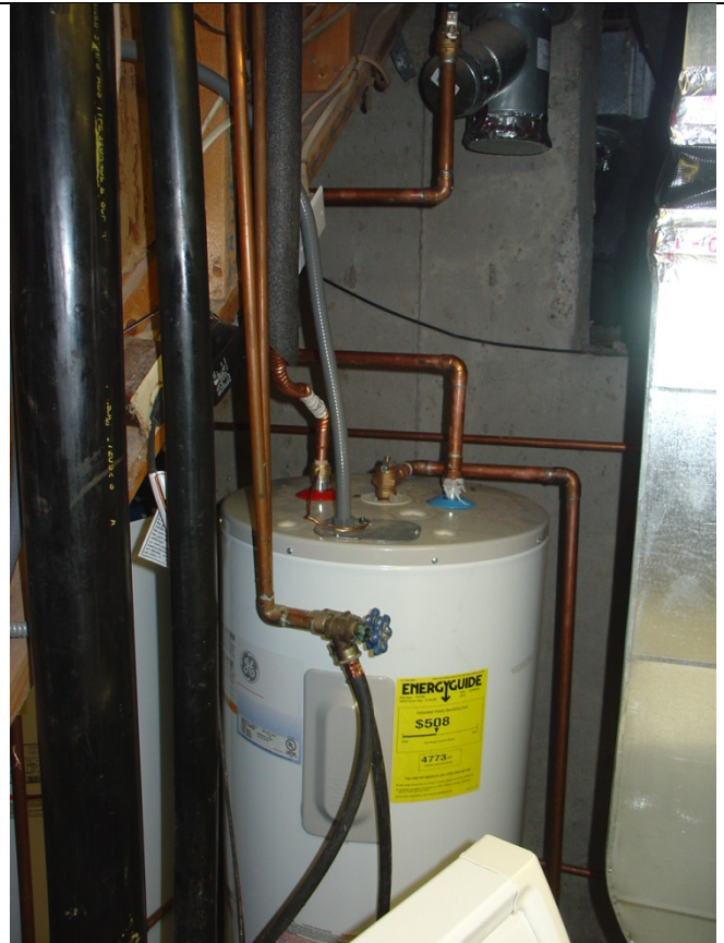
The Heat Pump system also preheats/heats water – a second preheat tank was tucked behind the primary electric hot water tank.
