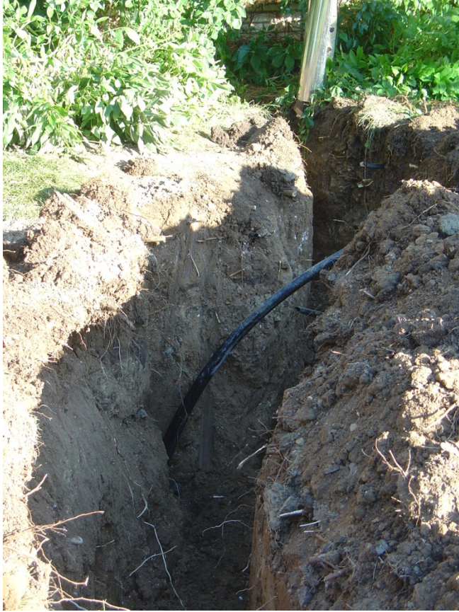
Ready to start connecting the two ground loops together
