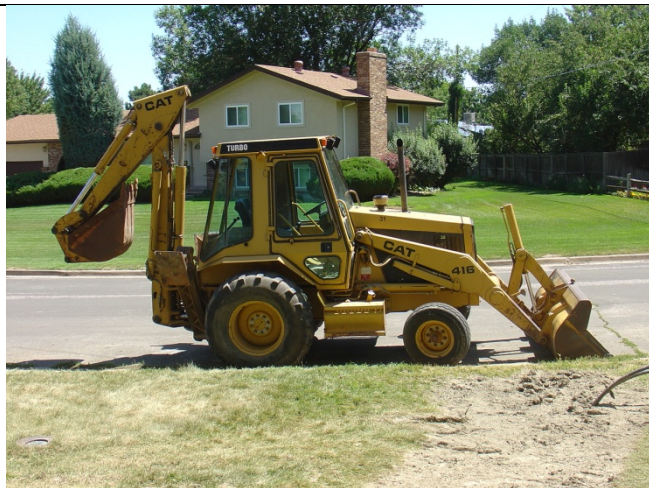
Are you ready for some trenching?
