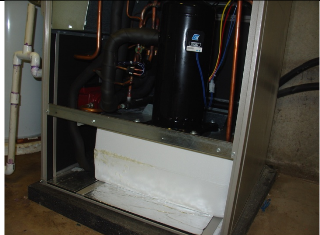
The ground loop coils are positioned just below the heat pump compressor (inside the styrofoam) for heat exchange with heat pump. No combustion anywhere – just the circulation of fluids that allow the house to exchange energy with earth – sustainably. No fossil fuel is consumed; zero emissions into the atmosphere.
