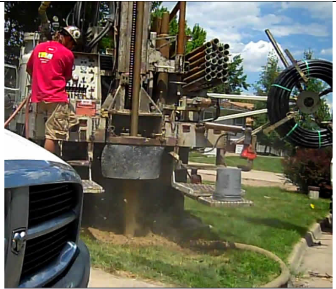
Drilling begins as high pressure water is forced into the drill pipe and out the lower end at the drill bit. The water is then forced back up the hole to emerge as a mud spray that impinges on the bottom of the platform (operator's knee level). The mud is then diverted by the black rubber shirt and falls back onto the ground around the hole. Notice the vacuum tube laying along the ground intended to vacuum up the emerging drilling mud.
