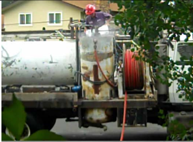
The operator of the grouting truck pours bags of thermal grout into the mixing chamber as they prepare a batch of grout (environmentally friendly bentonite clay).
