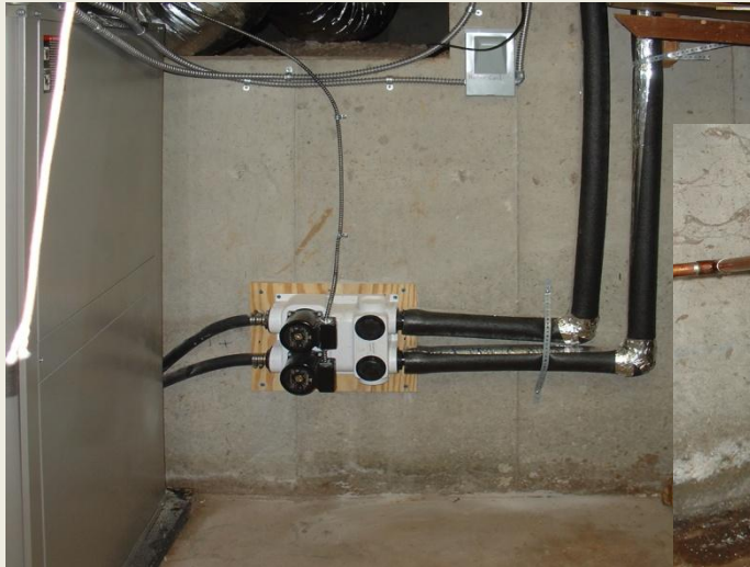
Ground Loop in basement with two circulation motors
