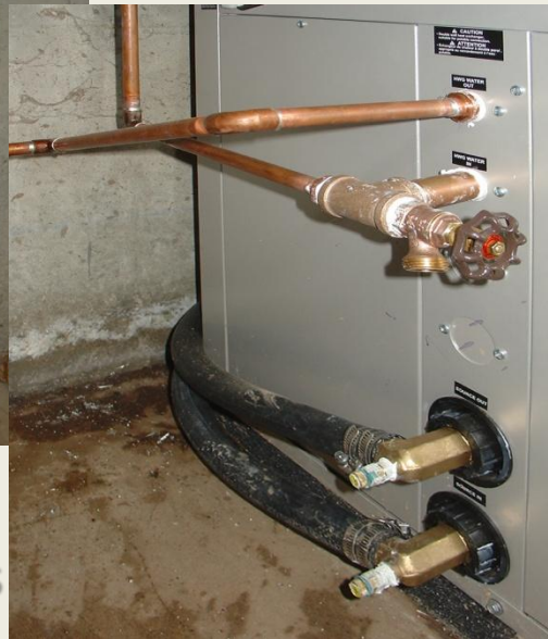
Connection of Ground Loop to Heat Pump
