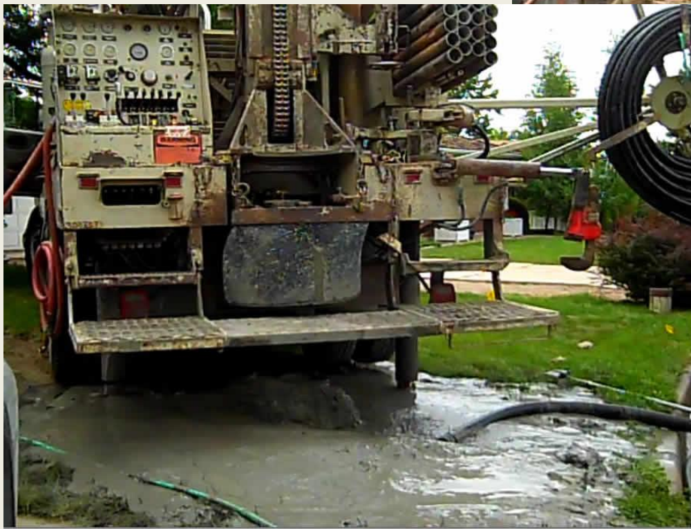
Drilling completed – now to suck up the mud
